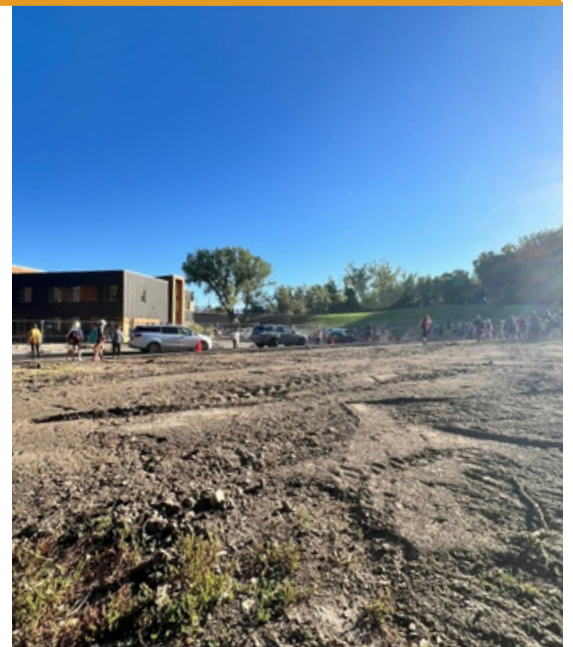
The first day of school looked a little different this year as our grounds have been prepped for change.
